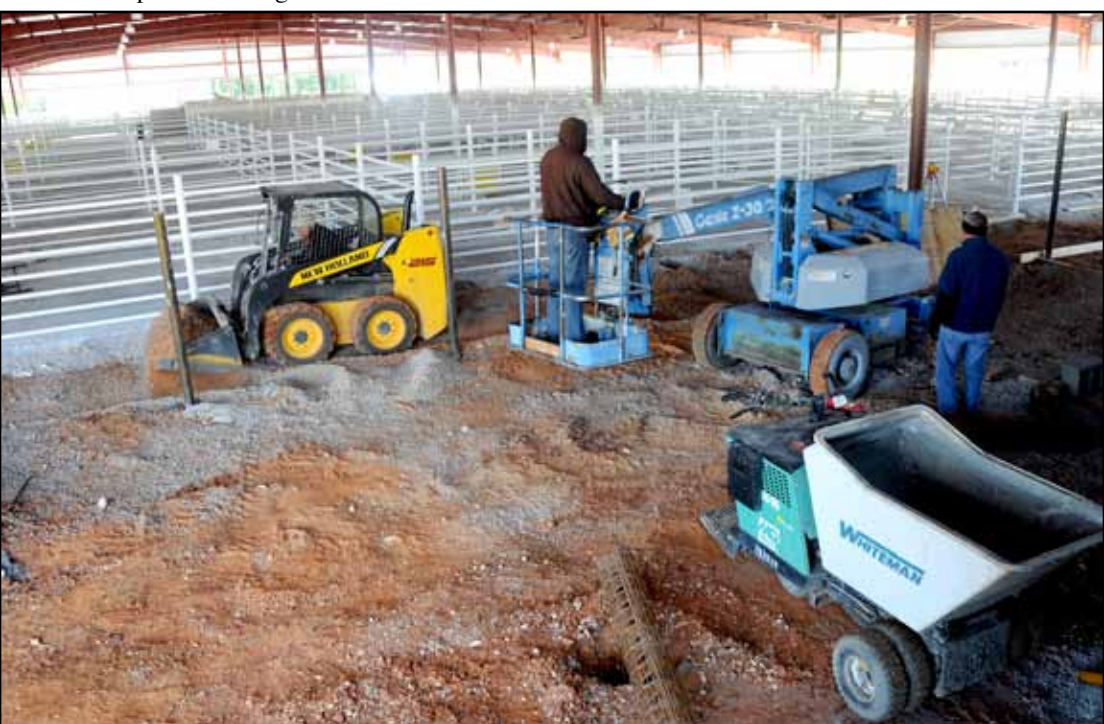
Above, construction workers welded pieces of metal together to form the outside portion of the gates that will house the cattle during sales. Below, workers were moving gravel and preping the area for concrete Monday. The area of the stockyards pictured below is where the cattle will be held during a sale. The area is around 54,000 square feet in size and is covered with a roof. The sides of the holding pins will be left open to allow good air flow.
