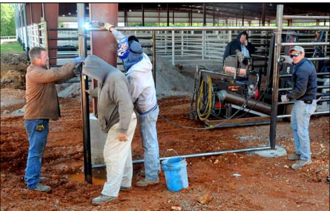
Above, construction workers welded pieces of metal together to form the outside portion of the gates that will house the cattle during sales. Below, workers were moving gravel and preping the area for concrete Monday. The area of the stockyards pictured below is where the cattle will be held during a sale. The area is around 54,000 square feet in size and is covered with a roof. The sides of the holding pins will be left open to allow good air flow.
